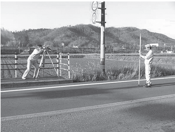
⑲高さ測量状況
